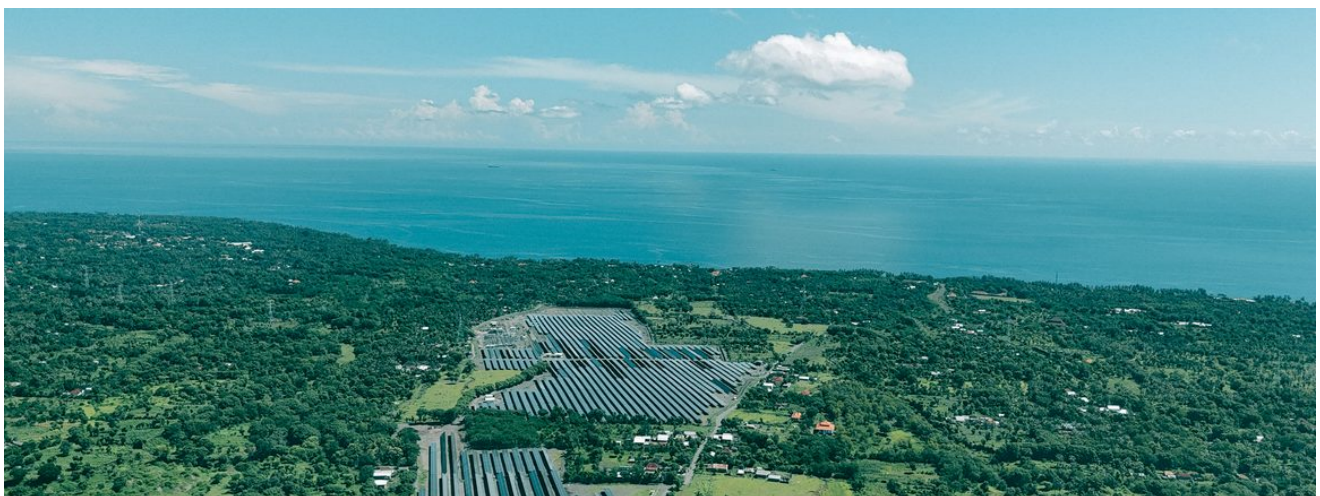
Island photovoltaic plant, a typical hybrid and off-grid configuration.
